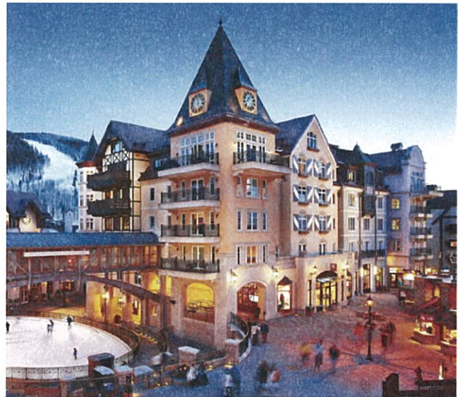
Image 31. Distinctive roof lines are created with roof forms and building heights that vary.
