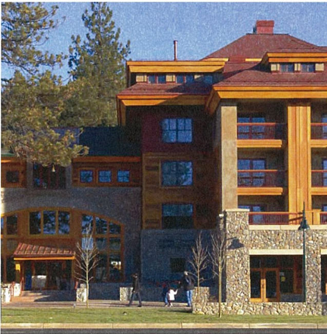
Image 28. Varying wall planes reduces the visual scale of a structure and helps to highlight interesting building features.
